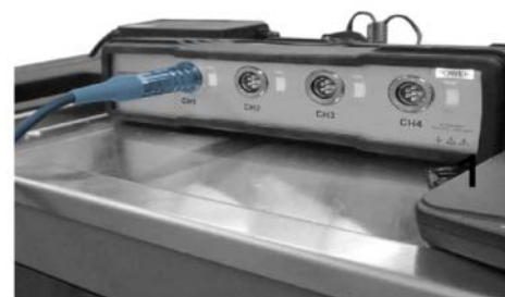
Connecting clamp-on ammeter to measurement and test equipment
