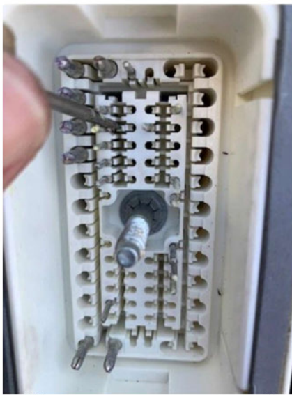
Fig. 9, Extracting the Terminal
