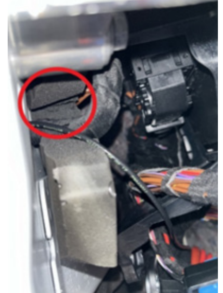
Figure 9 - Entry Point into Cavity (Foam Piece Circled)
