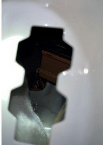
Figure 8 - Door Jam Internal Cavity
