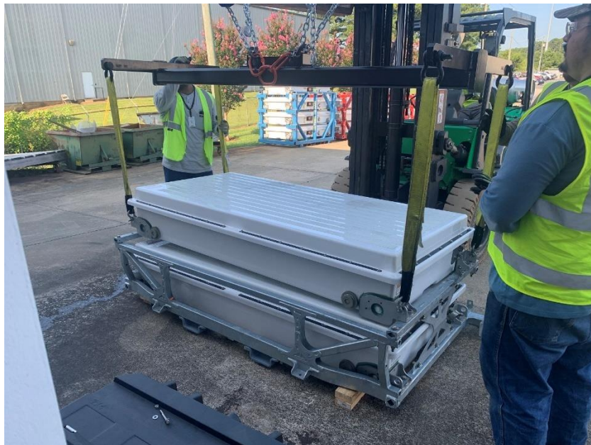
Figure 14: Rigging for lifting upper ESS battery pack.
