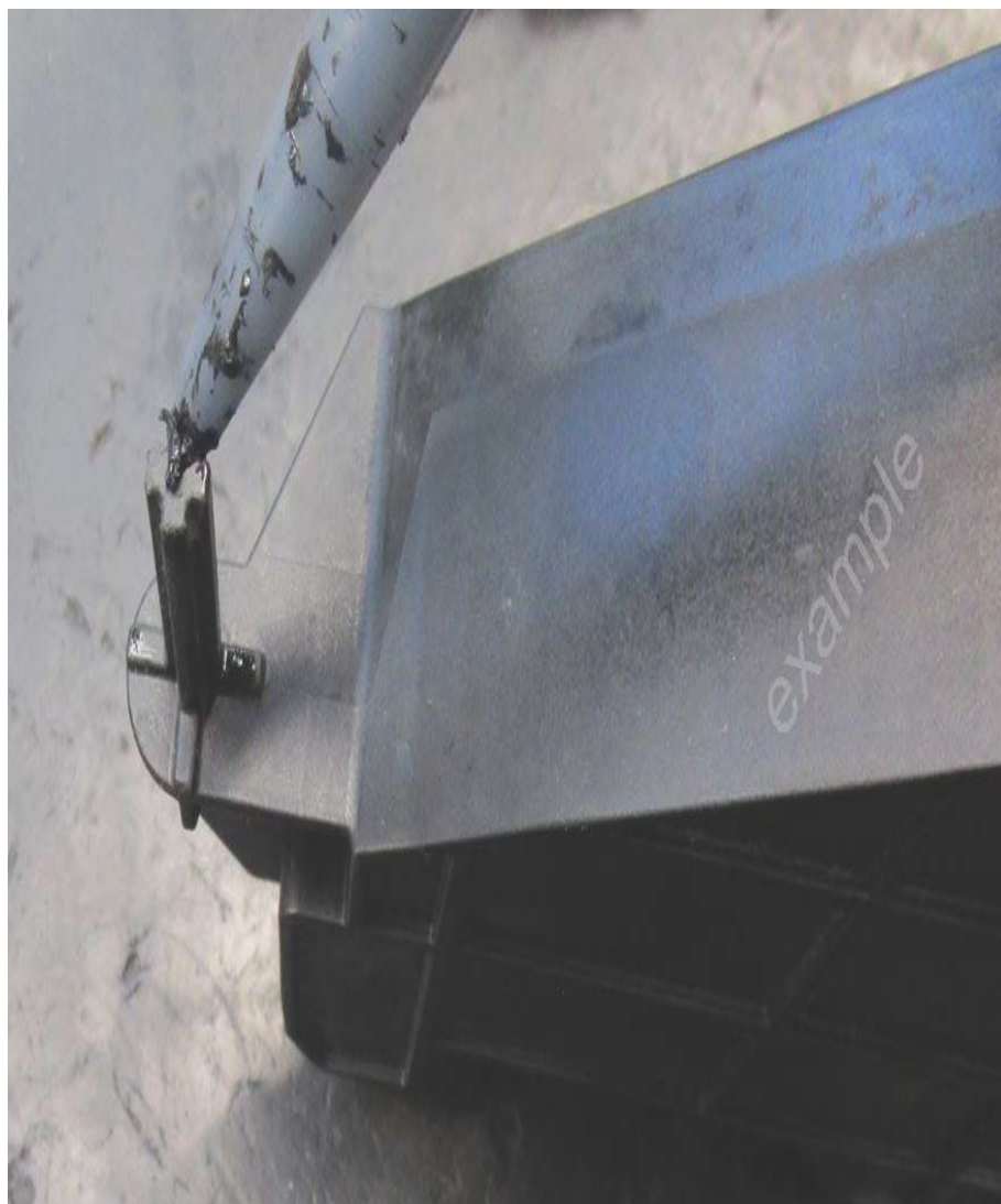
Figure 19. Lightly applying silicone sealant to attachment point (example).
