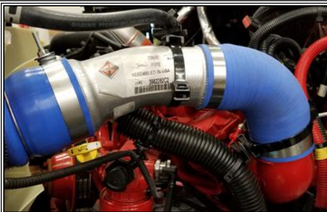
Figure 1: New CAC piping installed
