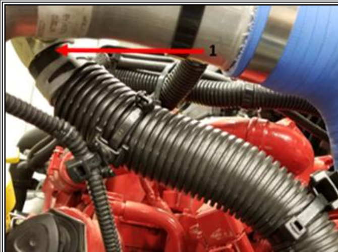
Figure 2: Air Compressor Inlet Hose
