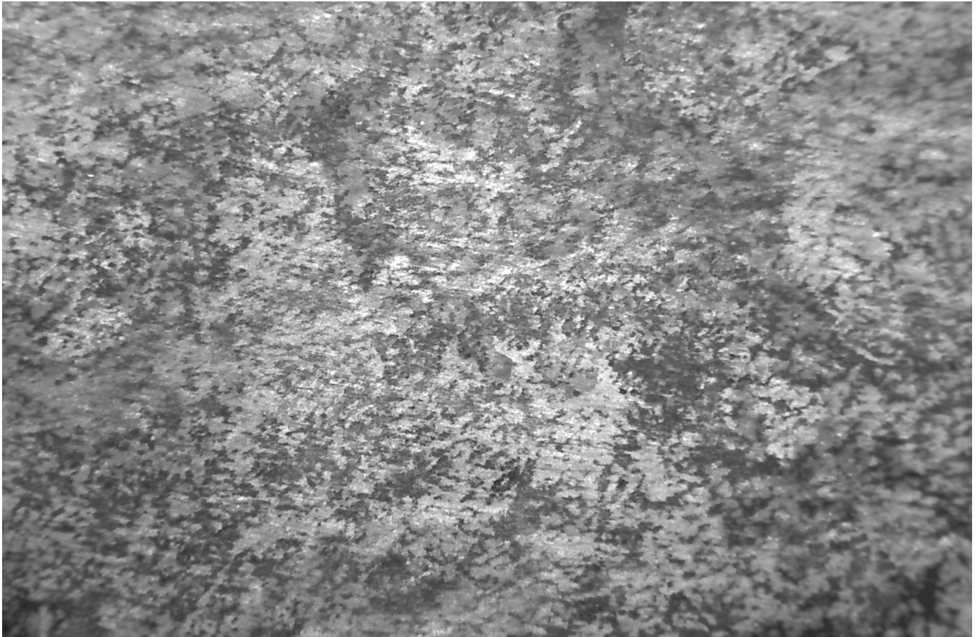
A close up of the sealing surface after cleaned with GM Low VOC Cleaner and plastic scraper.
