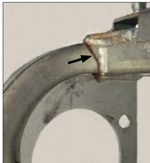
Figure 3 — Example of Crack in Tubing
