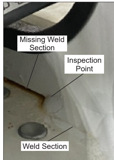
Figure 3 — Inside Side Plate Seam Inspection 1 of 2 Inspection points Pictured
