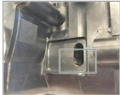
Slight traces of coolant (old type of coolant regulator without a leakage tank)
