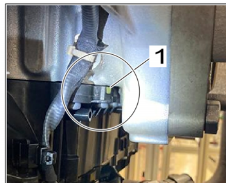
Oil leakage area
