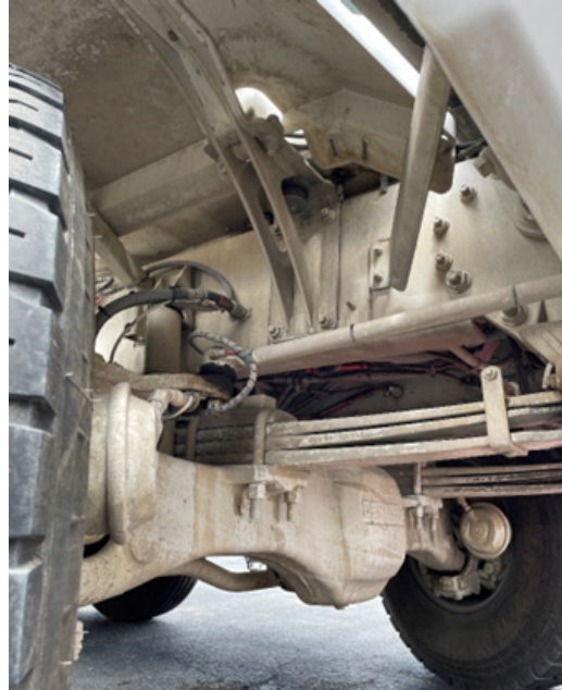
Access View with Front Wheels Turned Full Right
