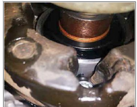
Oil leak on output-shaft radial shaft seal
