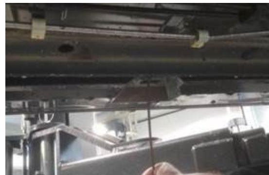
Figure 9. Making the hole in the sound absorber.
