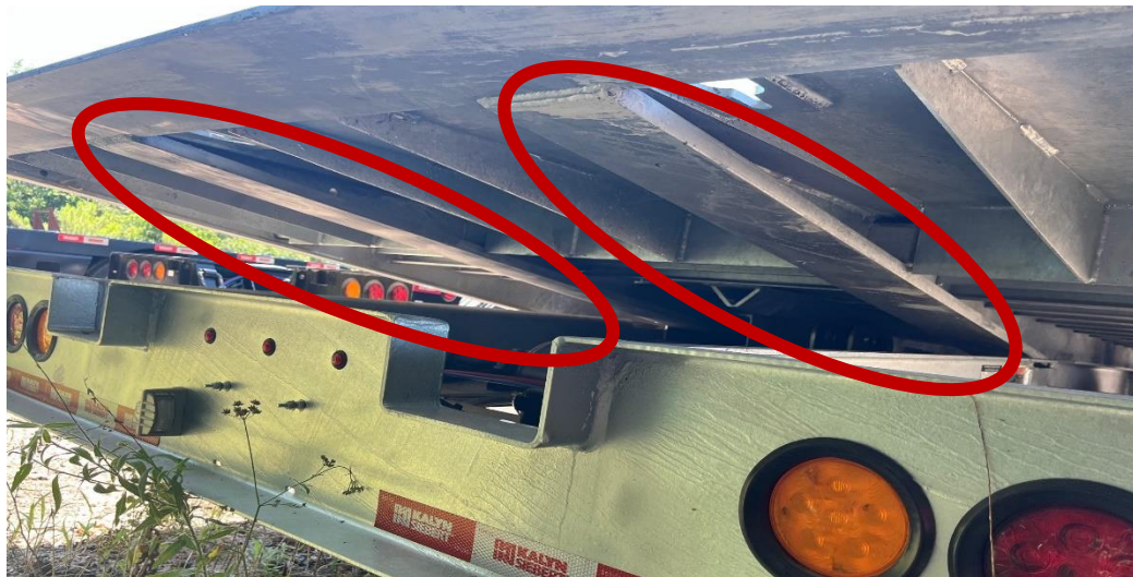
Main Beams underneath transition plate
