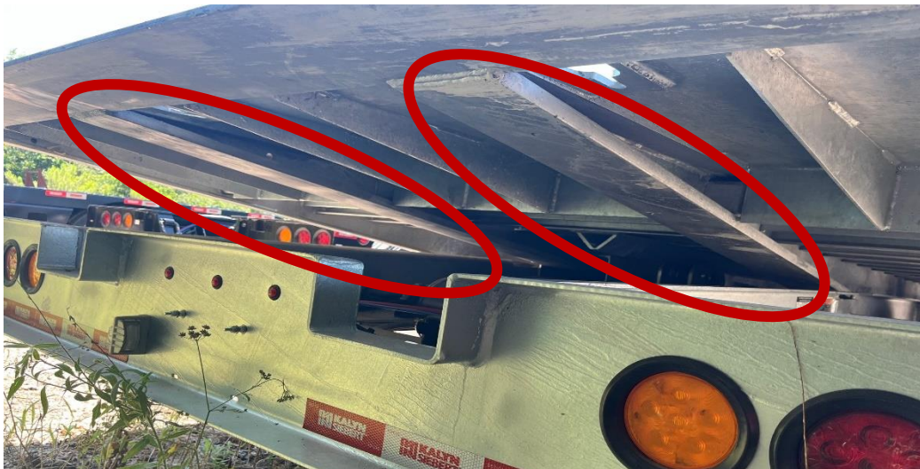
Main Beams underneath transition plate
