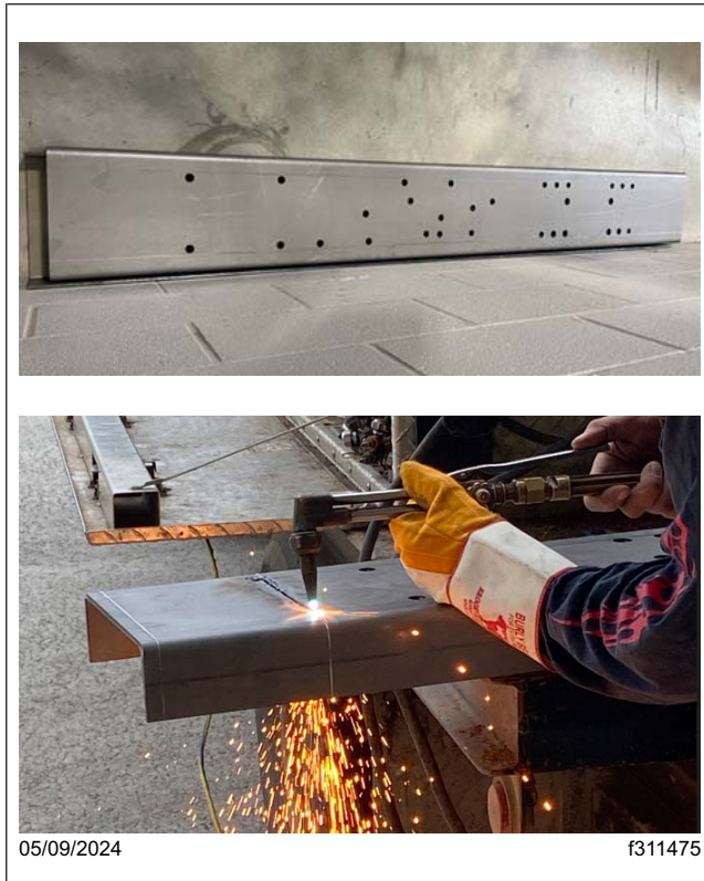
Fig. 33, Cutting the New Frame Rail to the Required Length
