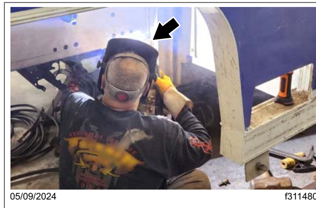
Fig. 38, Laying the Final Weld
