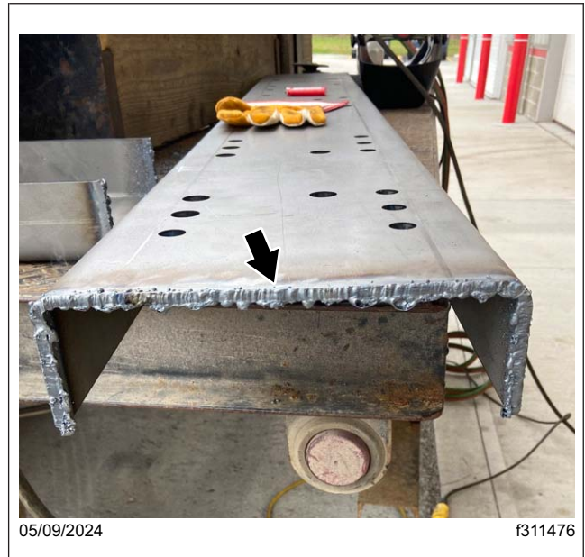
Fig. 34, New Frame Rail Cut to the Required Length
