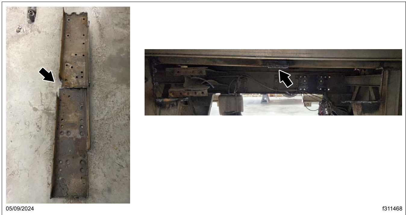
Fig. 27, Existing Welds on the Inside and Outside of the Frame Rail
