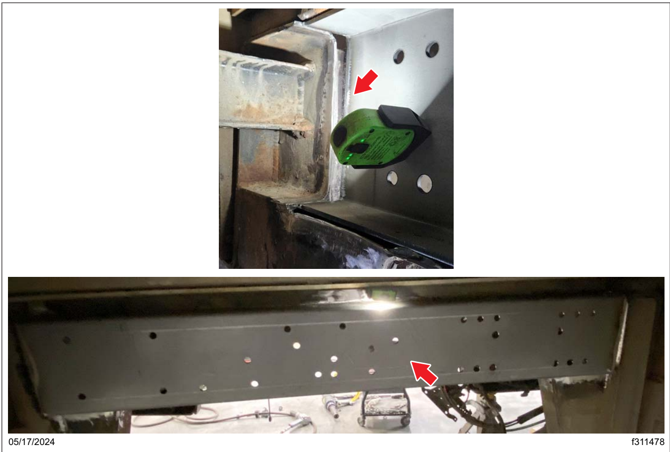
Fig. 36, Aligning the New Frame Rail
