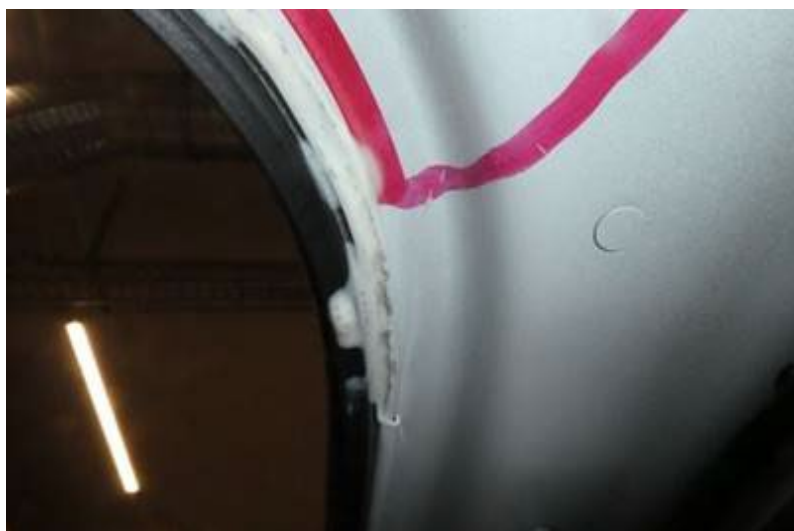
Figure 9. Gap created filled with Cavity Wax.
