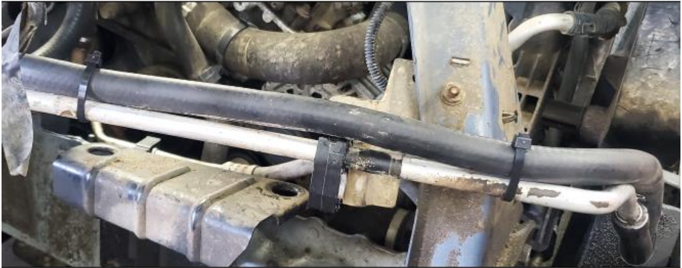
Cable ties used to secure routing of the repaired hose.
