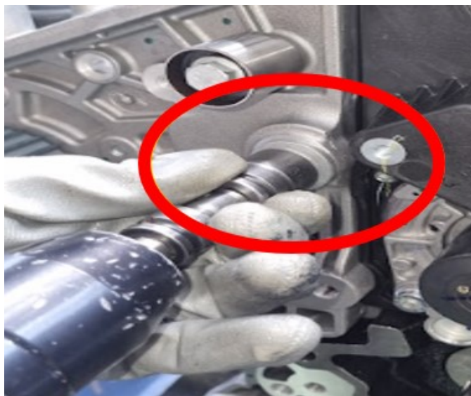
Fig. 4 Puma Bolt Tightening
