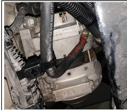
Fig. 4, Installation of Ground Cable at Lower Optional Ground Location
