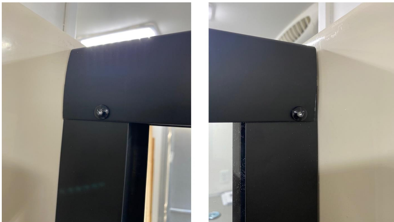
This is a split picture to show both ends of the shower top-rail with the added securement!
