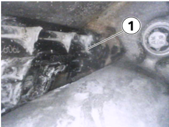
Coolant contamination on a fuel injector (1).
