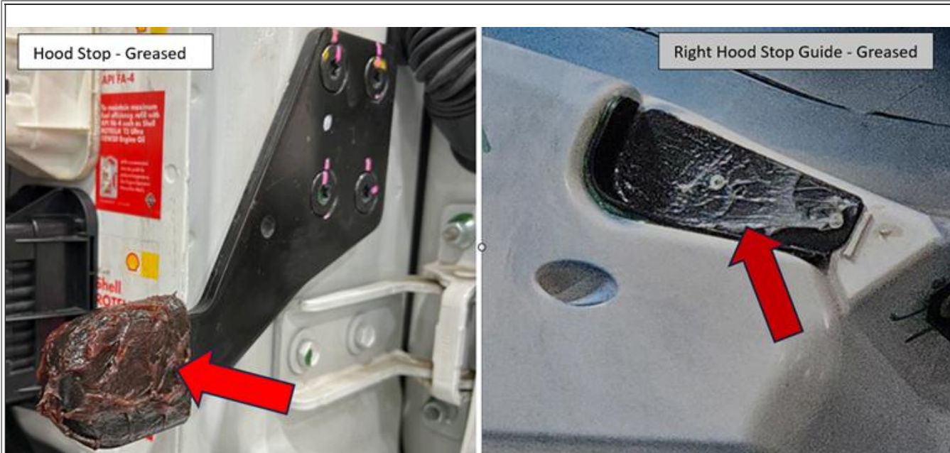
Figure 3: Newly added Grease to Hood Stops and Hood Guides
