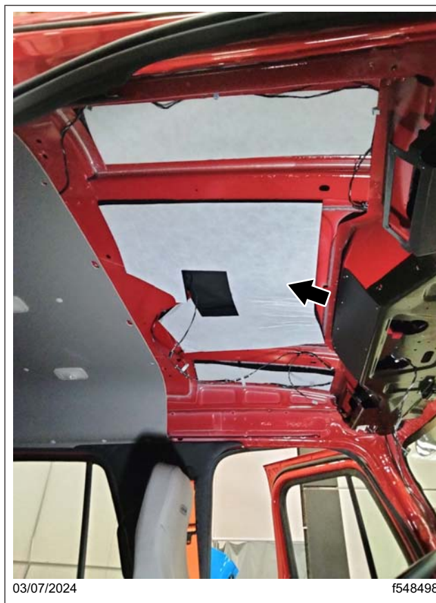
Fig. 2, Location of the Roof Insulation
