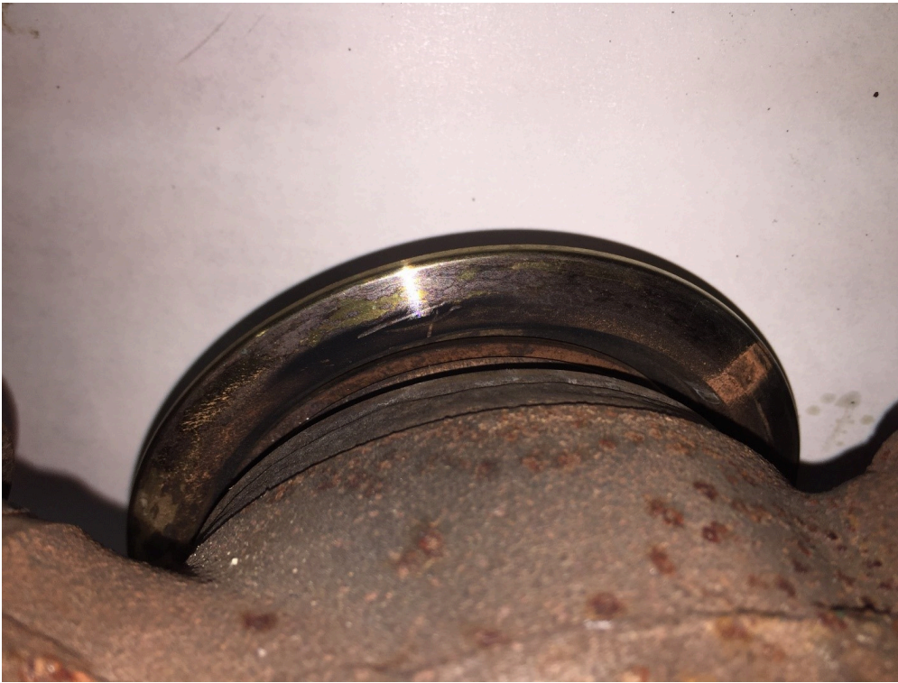
Flange weld at EGR cooler inlet
