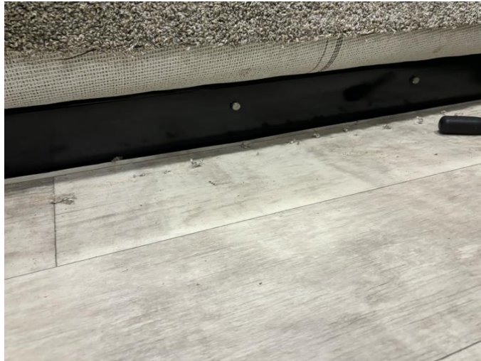
Single tube with lags with 3.5" lag bolt.
