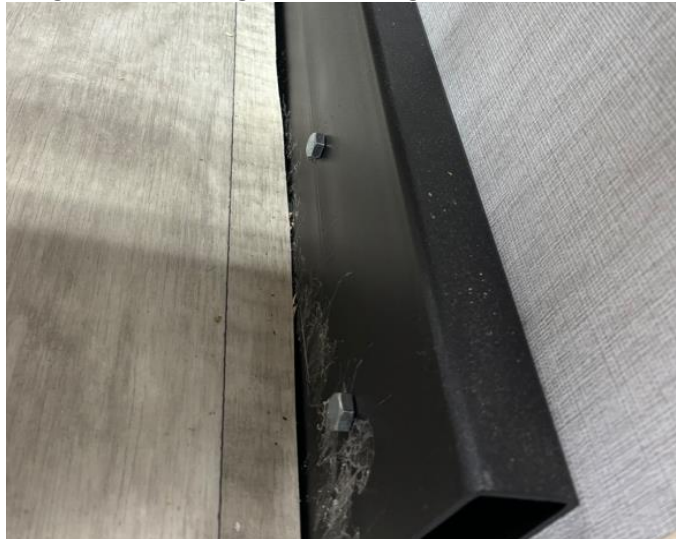
Single tube with lags with 3.5" lag bolt.
