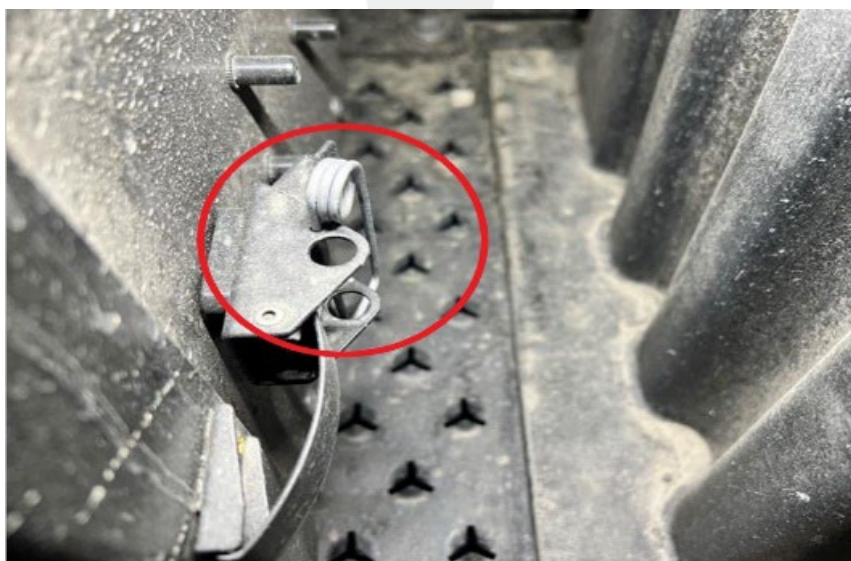
Figure 5 – Pin installed (4 total)
