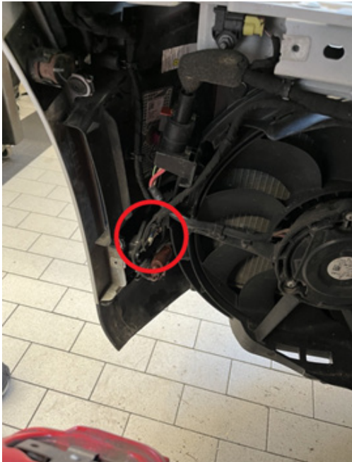
Figure 3 - Front Camera Connection Point (Front Driver Wheel Well)
