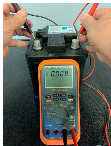
Figure 2 – Voltage test indicating an open connector
