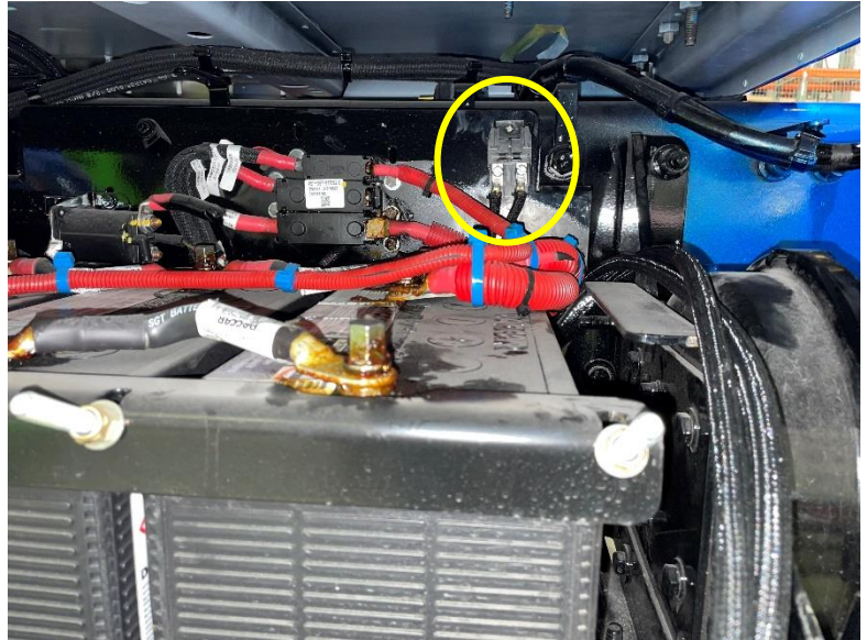
Figure 2: New fuse holder location
