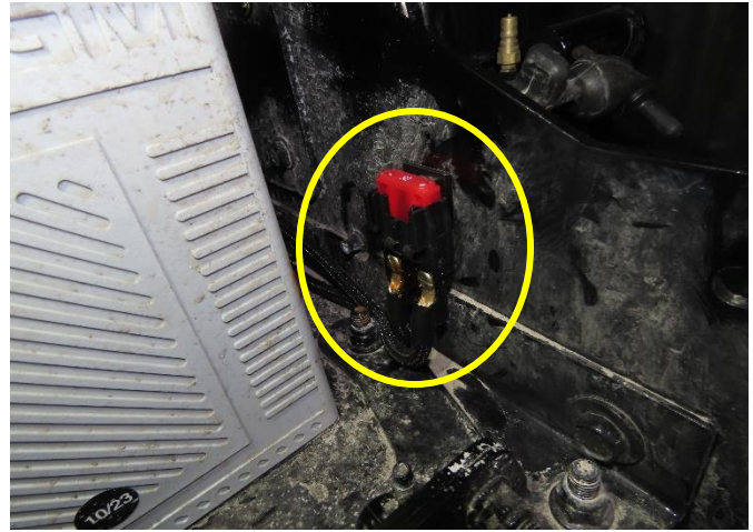
Figure 1: Current fuse holder location
