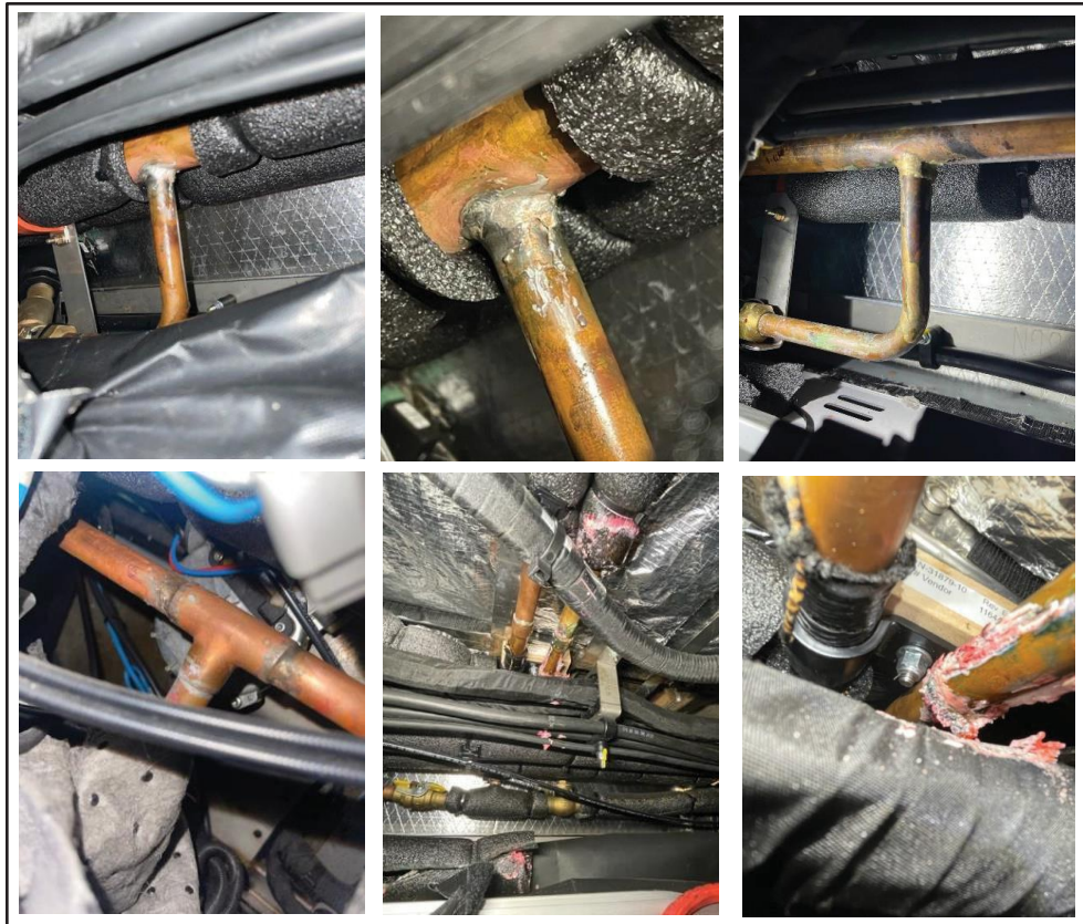
Figure 17 - Removal of Damaged Pipes
