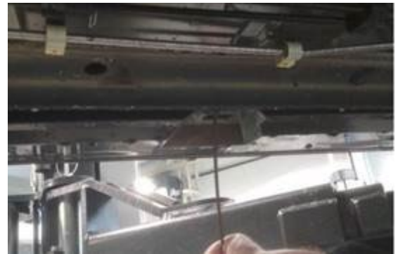
Figure 9. Making the hole in the sound absorber.
