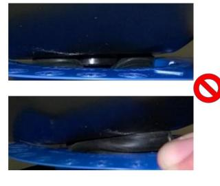
Incorrectly installed drain is shown.
