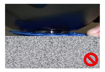
Incorrectly installed drain is shown.
