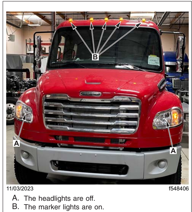
Fig. 97, Verifying the Headlights Turn Off and All Other Marker Lights Remain On After Turning On the Plow Light Switch
