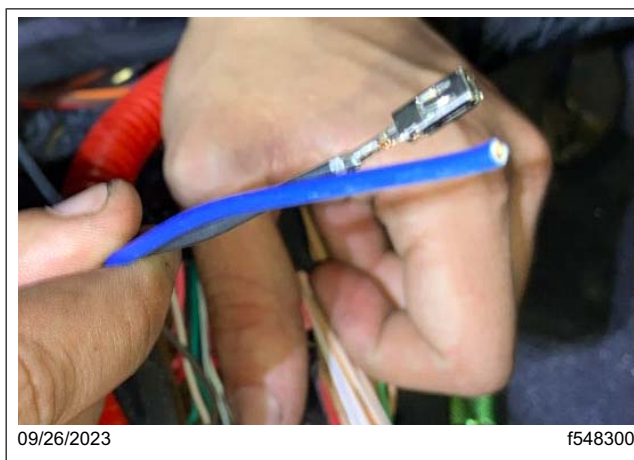
Fig. 32, Wire Removed from Cavity 6 of the SSAM X2 Connector and the Shorter Blue Wire, to be Spliced Together
