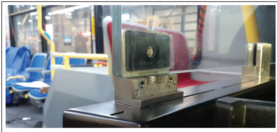
Figure 2 - Removal of Bottom Supports
