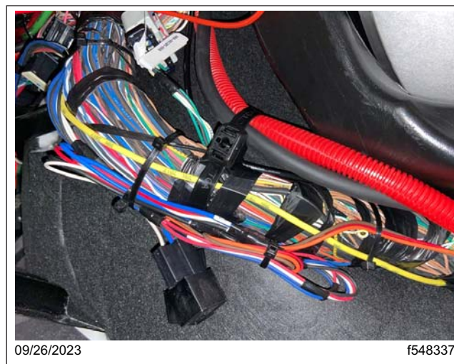
Fig. 69, Securing the Relays and Excess Wiring to the Main Harness Using Zip Ties
