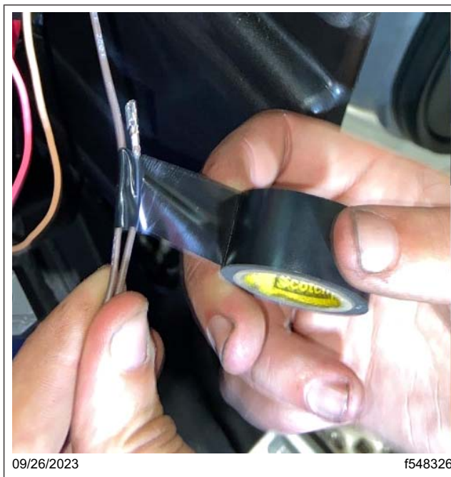
Fig. 58, Taping Up the Brown Wire
