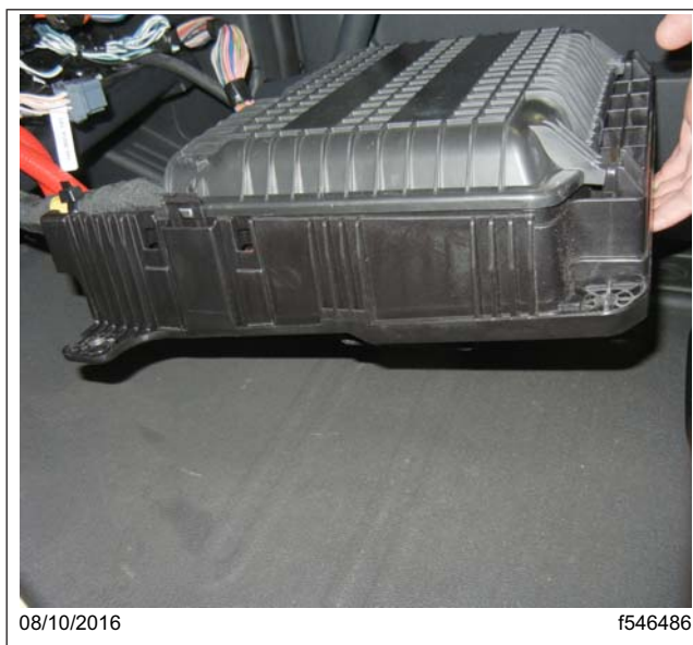
Fig. 27, Lowering the VPDM to the Cab Floor
