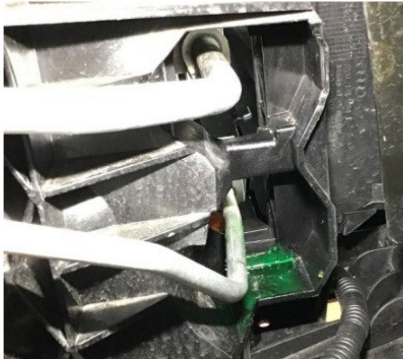
Figure 3. Evidence of a refrigerant leak with the seal strip removed.
