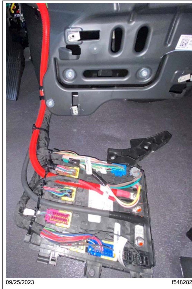
Fig. 14, SSAM Lowered to the Floor
