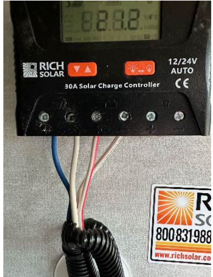
FIGURE 2 – CORRECTLY WIRED SOLAR CONTROLLER
