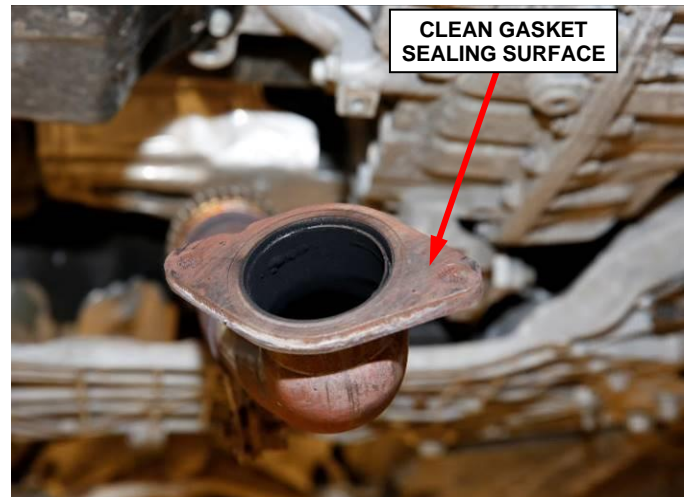
Figure 29 – Crossunder Pipe Flange
