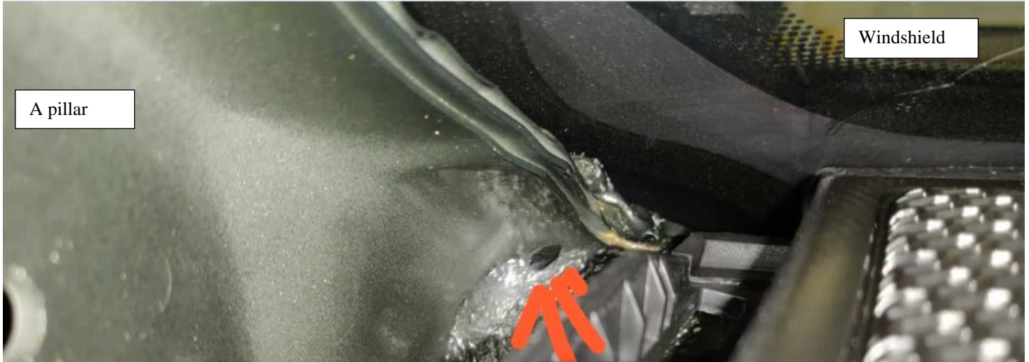
Example of a void in sealer viewed with A Pillar trim removed
