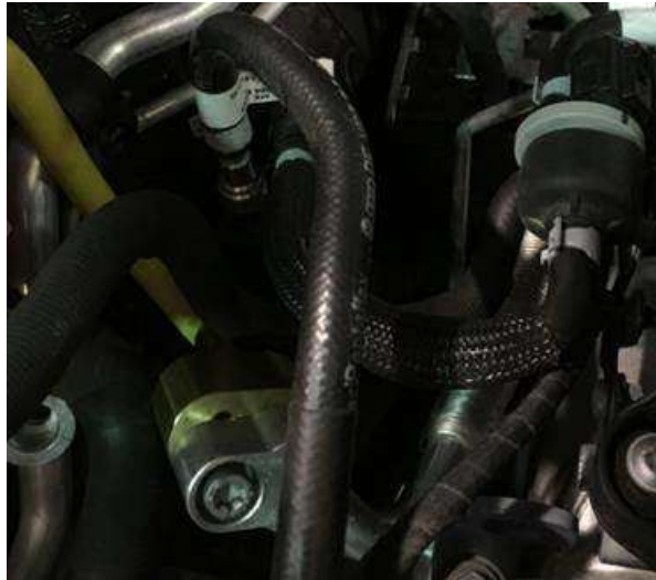
Figure 17. Attaching service station and flush hoses to rear A/C lines.
