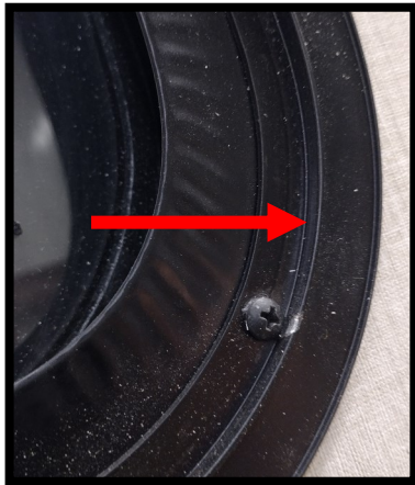
Fig 1 - INCORRECT installation - trim ring steps out away from the installer.
