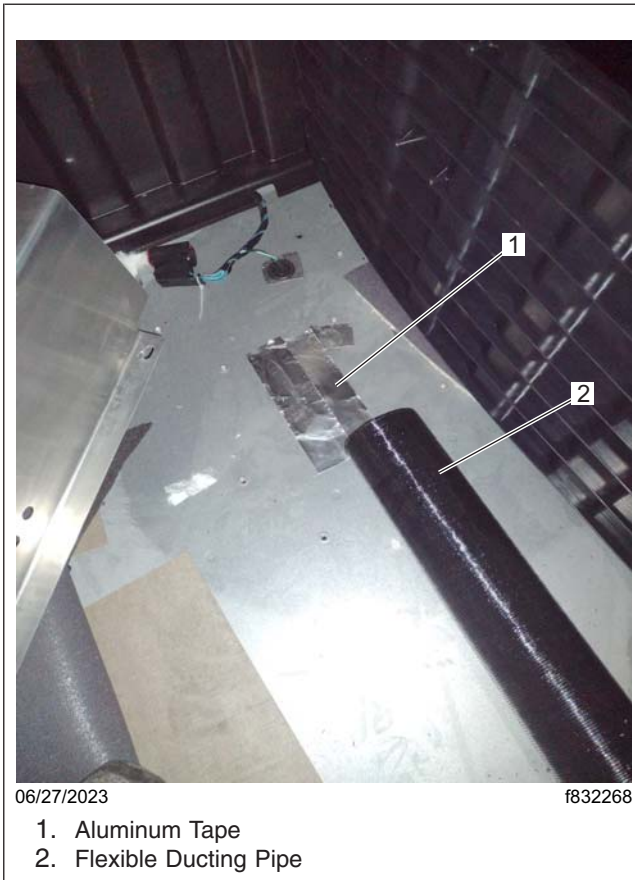
Fig. 3, Aluminum Tape Covering the Floor
