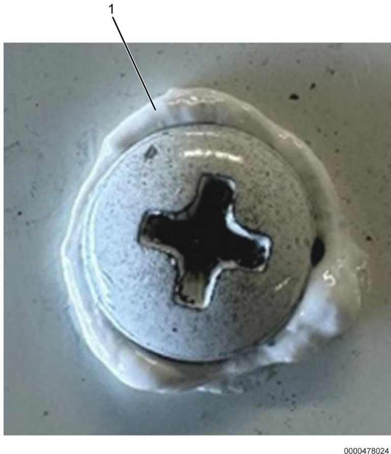
Figure 4. Add Sealant to Screws
