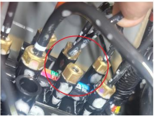
Check the air valves block pipes to ensure that there isn't any disconnected and/or wrongly installed line.
