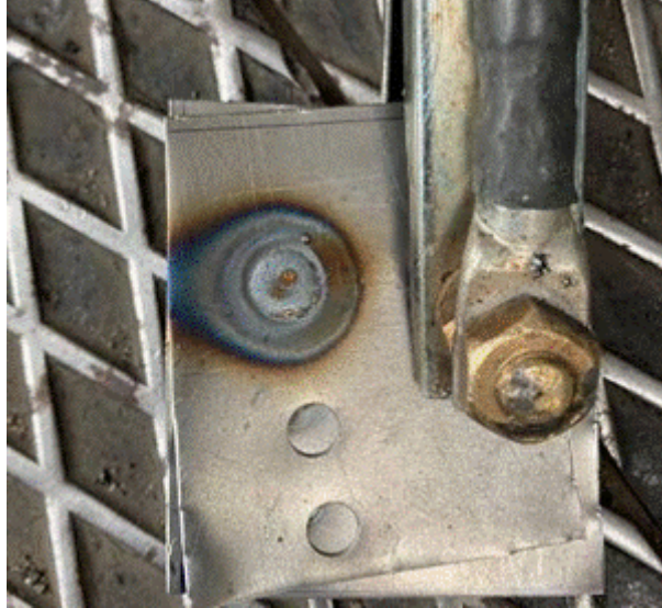
Figure 11. Performing a weld test.
