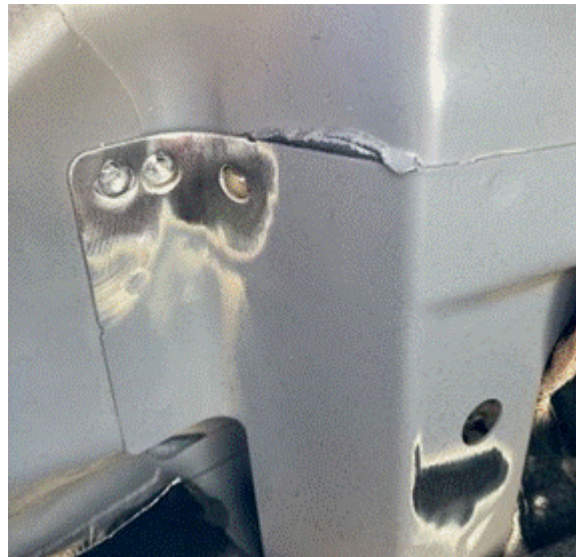
Figure 8. Surface prepared for welding.
