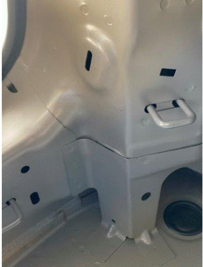
Figure 3. Area of left rear panel overlap to be repaired.
