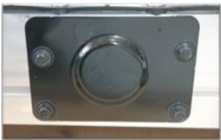
Image 3 – Vent Cap properly covered (Code 502)
