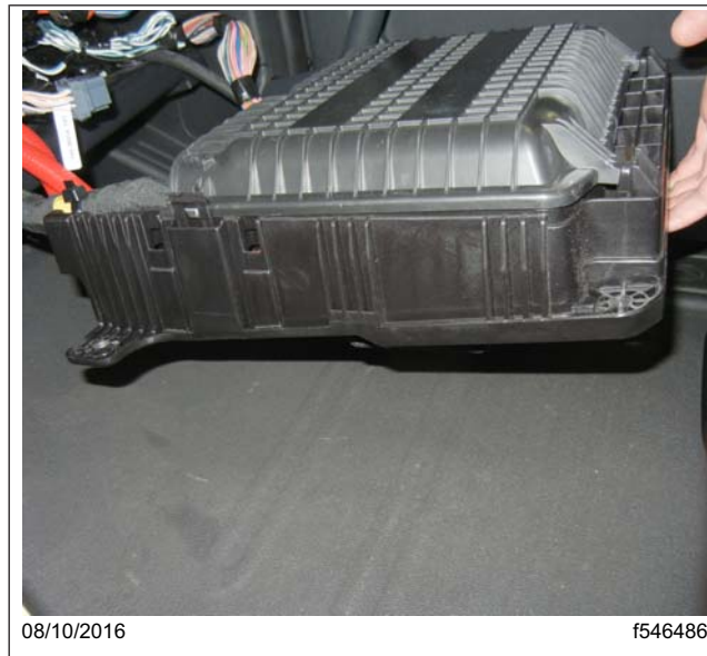
Fig. 27, Lowering the VPDM to the Cab Floor
